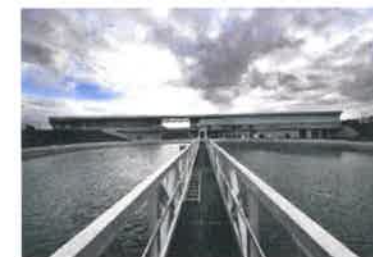
Figure 13 - Station d'épuration - Mainvilliers
